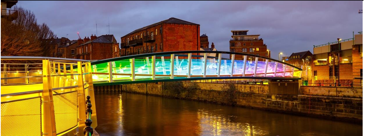
Completed David Oluwale Bridge illuminated at night over the River Aire, connecting Sovereign Street and Water Lane
