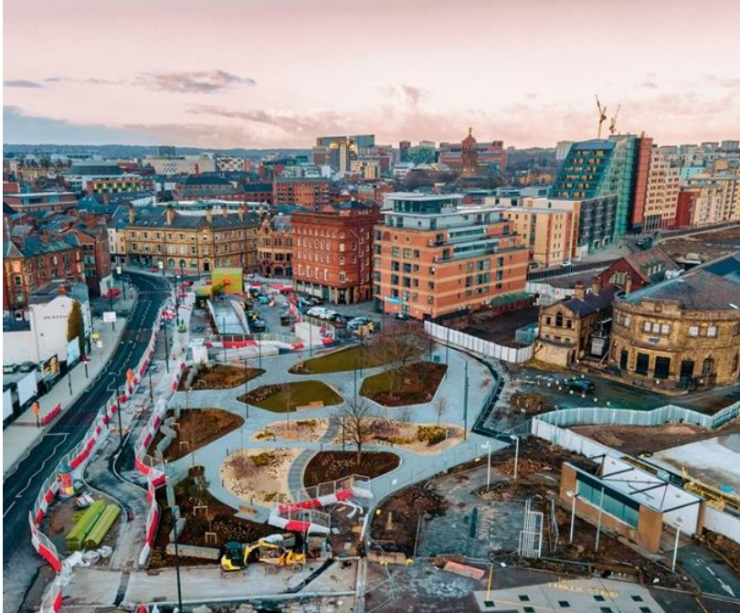
Section of the City Centre park nearing completion on Meadow Lane, part of the wider Aire Park development
